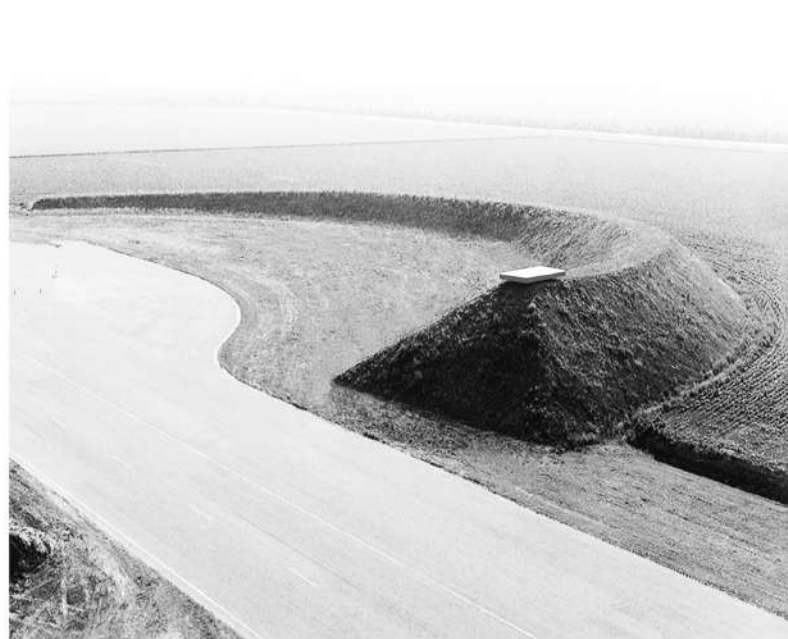
Sx: Protection structures against snow avalanches in Siglufjordur, Landslag, 1998-1999 Dx: Homage to El Lissitzki, Lelystad, 1985-1986
