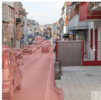
1 Busy SS16 with very narrow road section. Absence of sidewalk in some portions.
