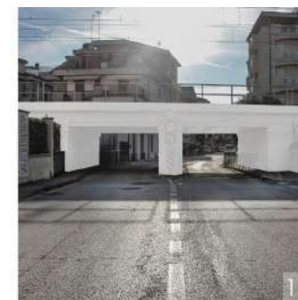
11 One of the three subway connecting the Waterfront, on Voltattorni Street.
