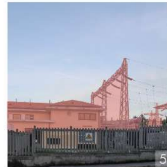
5 Electrical substation, close to schools and visual interference element.
