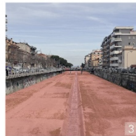
3 Albua stream completely cemented, does not allow water absorption in case of flooding.
