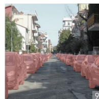
9 Via Monte San Michele, an important historical axis, unmaintained, has parking on both sides and almost no sidewalks.
